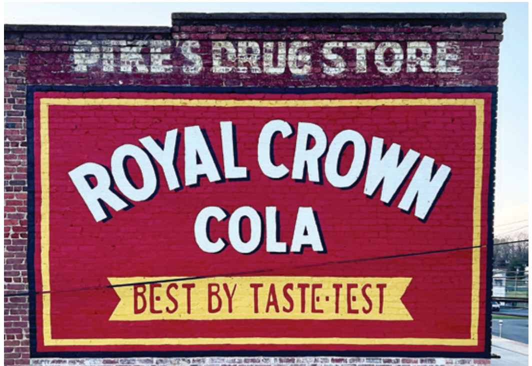
The Royal Crown Cola restoration in Oakboro was completed in March 2023.
